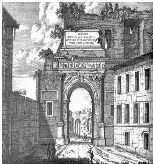
Fig 2. Detail from a plate portraying Rome's palaces and ruins and even reconstruction of ancient buildings in Rome. The second states of these etchings were collected in the publication by Peter Schenck (1660-1711): 'Roma aeterna, sive ipsius aedificiorum Romanorum, integrorum collapsorumque, conspectus duplex.' In the 'Aedificiorum Index': '16. Arcus Imperatoris Titi Vespasiani', view on the Arch of Vespasianus. Inscribed on the bottom in Latin: 'ARCUS Imperatoris TITI VESPASIANI Temporis hostiumque favite foede mutilatus.' (Detail from "Enciclopedia di Roma" [16]. For the history of the Arch see the note b, in the text.
